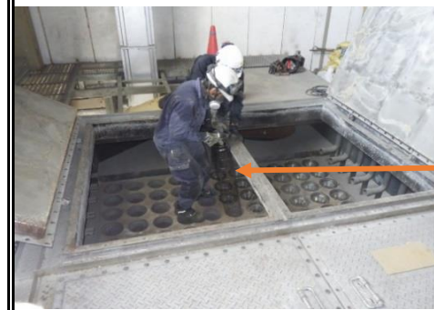
ろ過式集じん器上部点検口③
